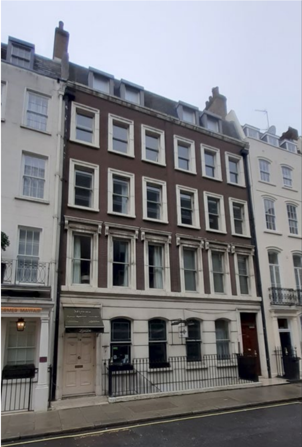
Front Elevation of the Building:
